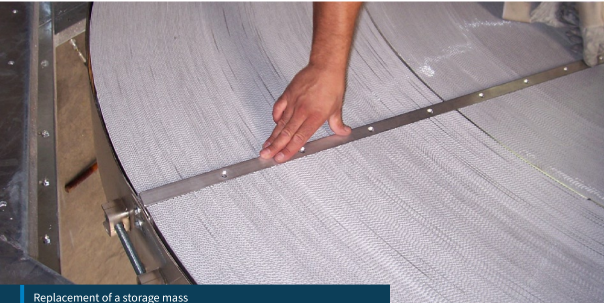
Replacement of a storage mass
